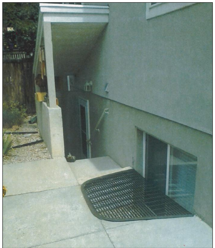
West Façade with Basement Entrance
